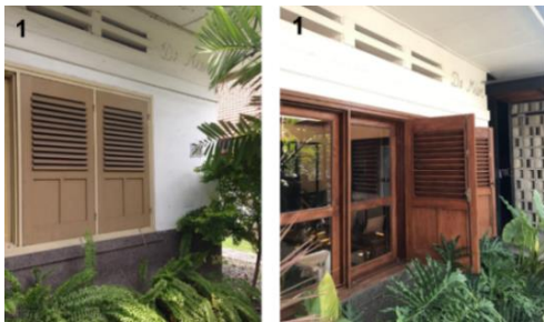
Figure 9. The front window is conserved before (left) and after (right). Source: Spasi Architects' documentation and author's documentation, 2022
