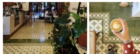
Figure 6. Main building tile after conservation.
