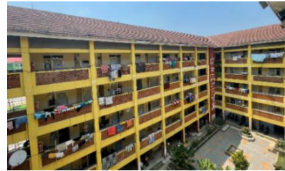
Gambar 4. Courtyard Rusunawa Cingised Blok 4
